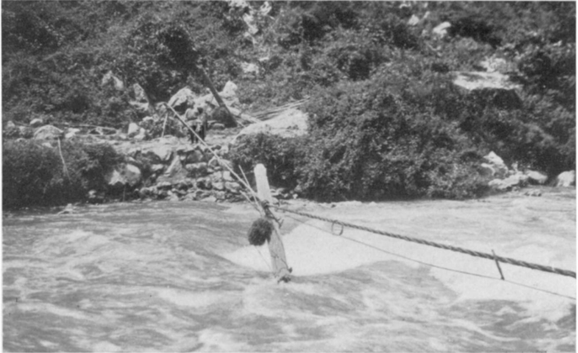
FIG. 13—A type of rope bridge for goods and passengers in common use in the tribes country.
