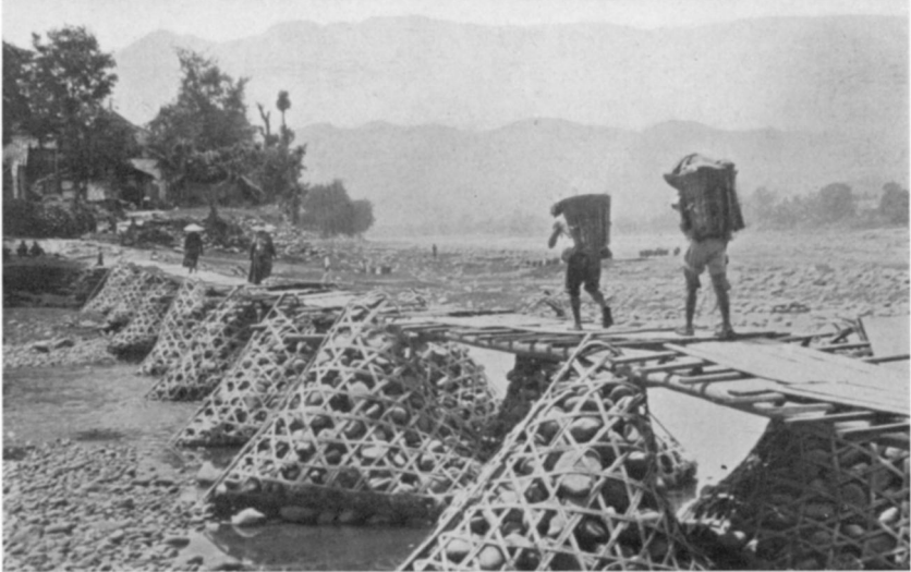
FIG. 12—Stone basket bridge near Yachow. The bridge is replaced yearly after floods.
